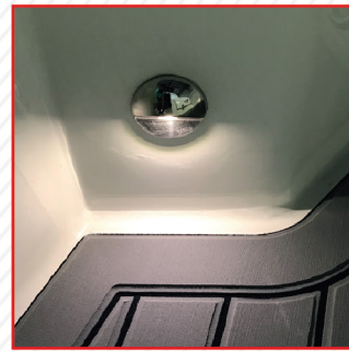
LED floor lighting
